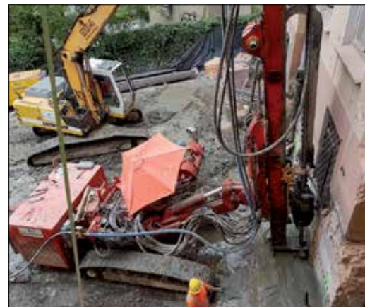
Fot. 6 | Prace – jet grouting
