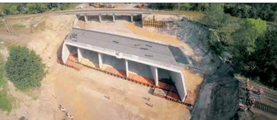
Fot. 6 | Transport tunelu TK-2
