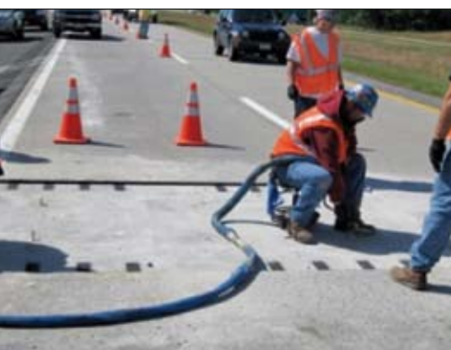
Fot. 1 | Wtłaczanie zaczynu cementowego ( http://precast.org/2011/05/precast-concrete-paving-slabs-built-to-last-and-install-fast )
