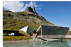
Norwegian Tourist Route service building at Trollstigen, equipped with a Jets™ system.
