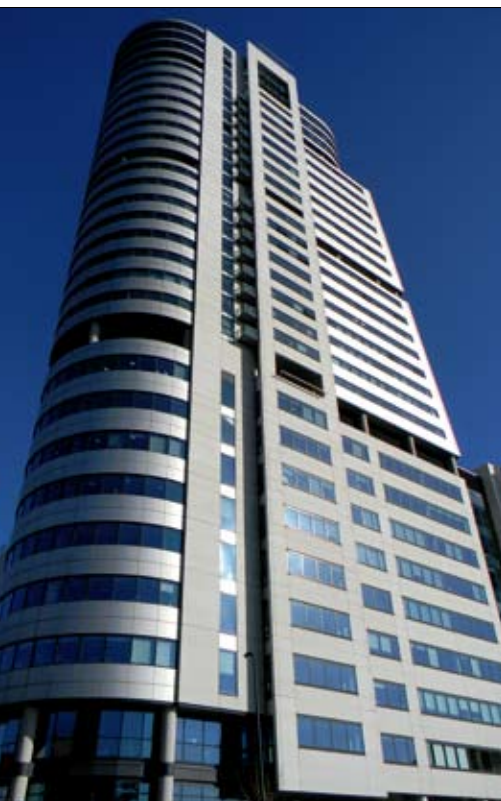
Fot. 2 | Bridgewater Place w Leeds (fot. Lad 2011, Wikipedia)
