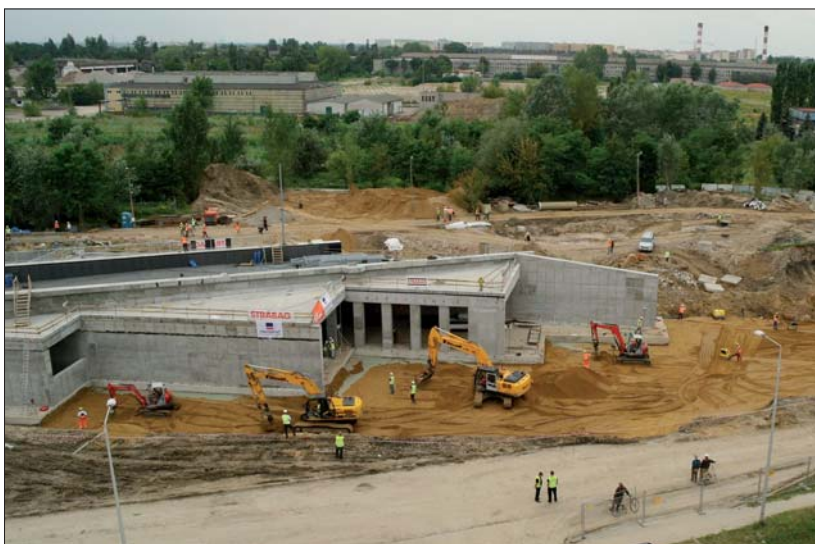
Fot. 9 | Nasuwka tunelu
